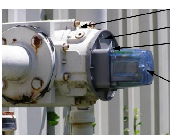
TCI Installed on a Rotary Meter
